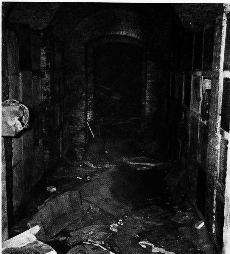
Fig. 25. The Interior of the Main Catacomb, showing damage caused by vandals. The long barrel-vault and cross-barrel-vaults can be seen (Photograph by Ian Williams, kindly provided by the London Borough of Southwark.)
