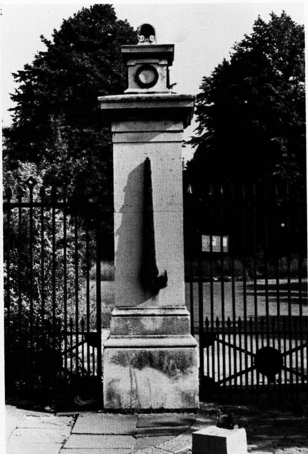
Fig. 19. Detail of one of the Portland Stone gate piers, designed by J. B. Bunning, and erected in 1840. The assured classical detailing, with inverted cast iron torch, demonstrates Bunning's skill as a designer. The Serpent eating its own tail on the die of the pedestal is symbolic of eternity. (Photograph of 1976 by James Stevens Curl.)
